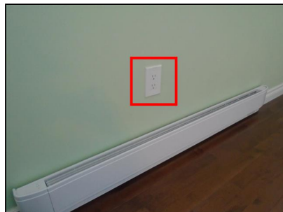
6.3 Item 8(Picture) Multiple receptacles throughout top floor
