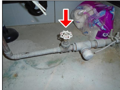
8.4 Item 1(Picture) Bathroom closet
