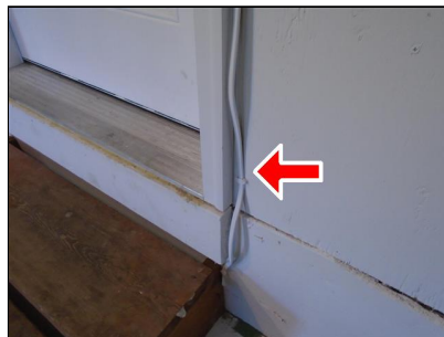
6.2 Item 3(Picture) Garage
