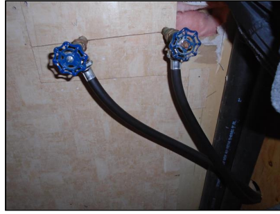
8.1 Item 3(Picture) Rubber hoses
