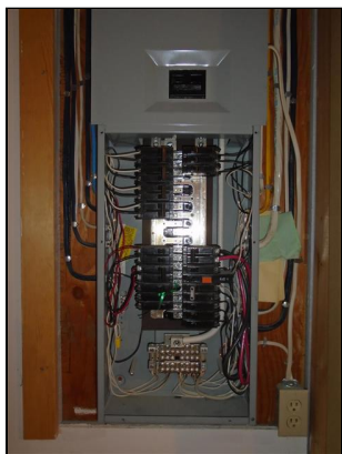
6.7 Item 1(Picture) Main (Southeast corner)
