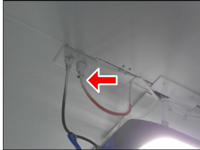
6.3 Item 2(Picture) Garage
