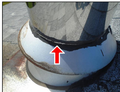
2.2 Item 1(Picture) Metal chimney
