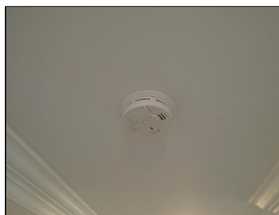
6.8 Item 1(Picture) Only one found in the upstairs hallway
