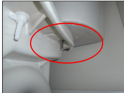
8.2 Item 1(Picture) Basement
