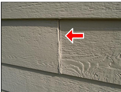
1.0 Item 1(Picture) South side
