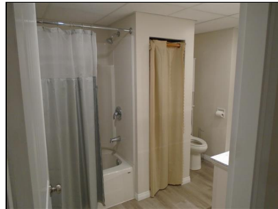
4.4 Item 5(Picture) Basement
