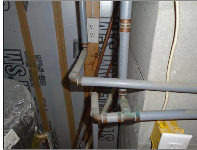
8.1 Item 1(Picture) Basement
