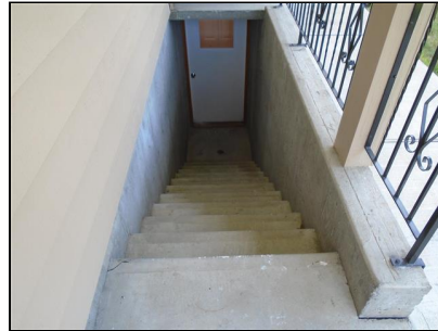
1.3 Item 8(Picture) Basement entrance
