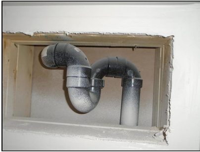
8.0 Item 2(Picture) Basement laundry
