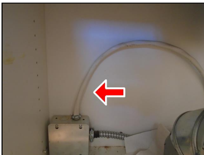
6.2 Item 2(Picture) Under kitchen stove
